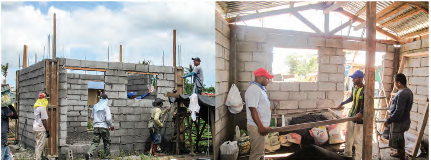
Brothers constructing housing unit in Brgy. Caroyroyan, Pili.
