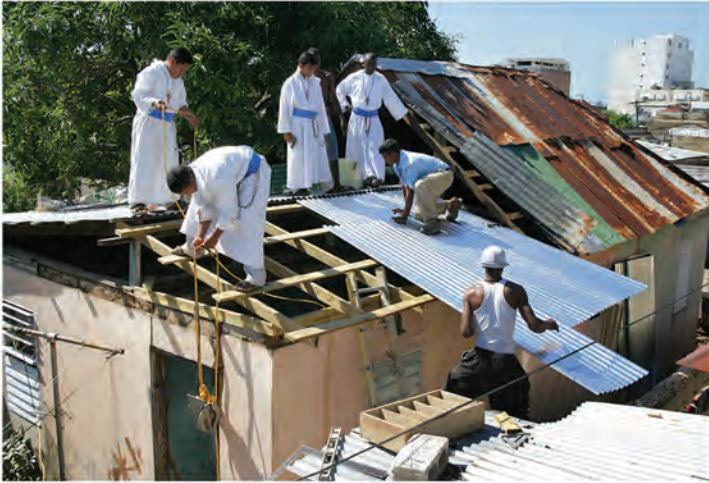
Brothers fixing dilapidated house.
